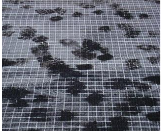
Figure 8 : Foot marks visible on Glasstex immediately after installation over bond coat
