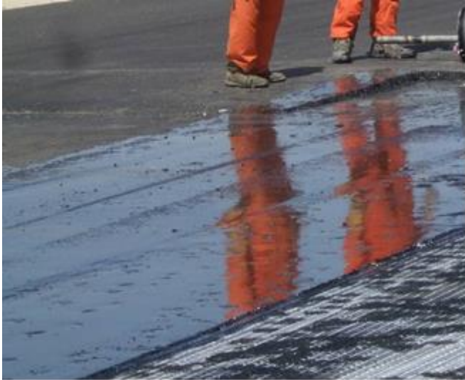
Figure 7 : Mirror effect of bond coat immediately after application
